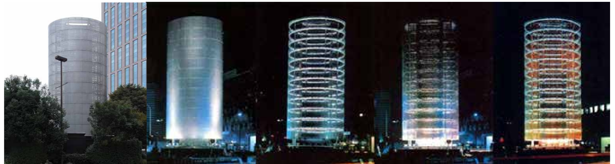
Tower of winds, Toyo Ito, Yokohama, Japan
