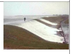
As part of the Future Flood Risk Management Technologies project, we plan to build a large-scale experimental setup at the Delft University of Technology to study the flow characteristics of an overtopping wave (see figure below). These unique experiments allow to study the overtopping flow on a 3 to 4 meter high slope. Currently, we are preparing the experimental setup and aim to start these experiments around April 2025.
